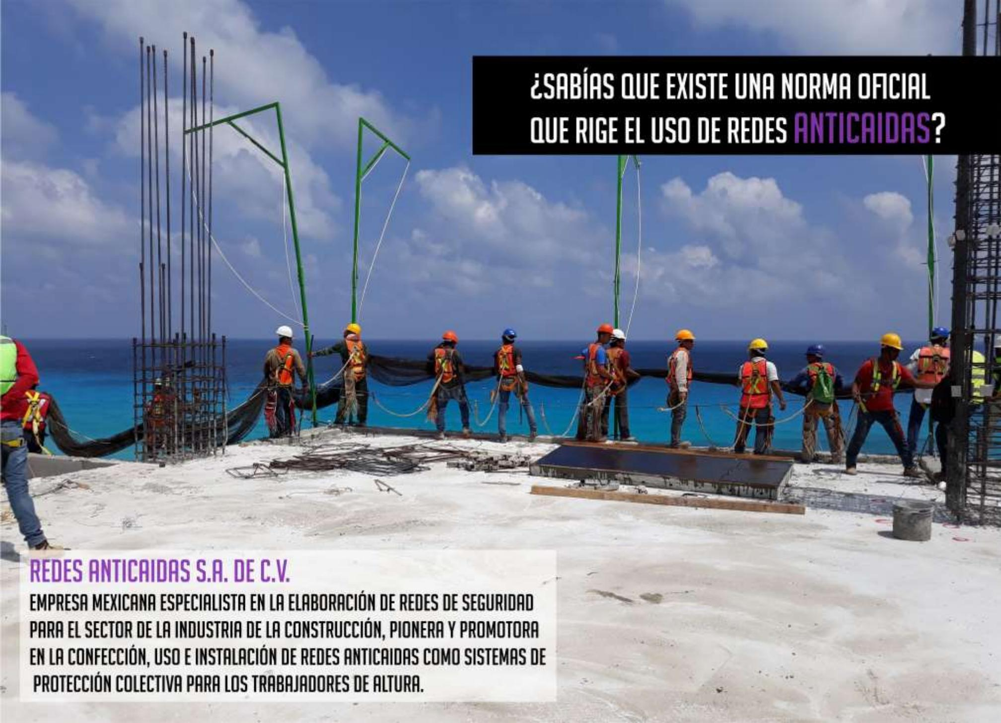
A group of construction workers in safety gear are working on a high-rise building. They are holding up a large black safety net that is being attached to a green metal frame. The workers are standing on a concrete floor with rebar structures. In the background, there is a clear blue sky and a view of the ocean. The overall scene is a busy construction site.
